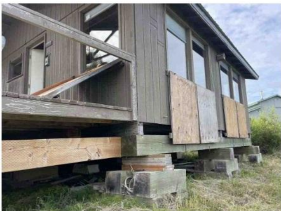
North Cabin Side
