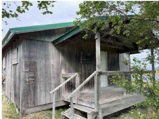
South Cabin Front
