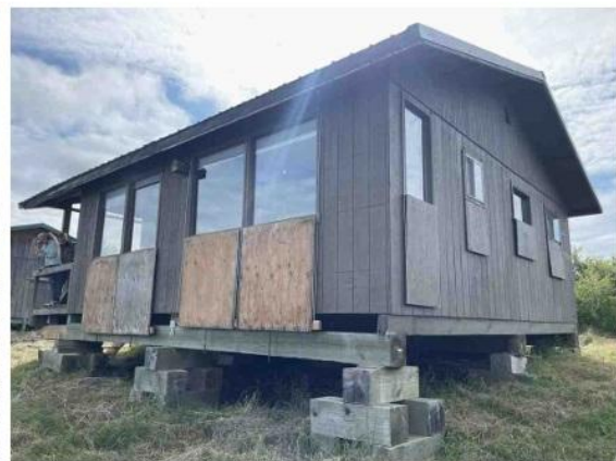
North Cabin Rear
